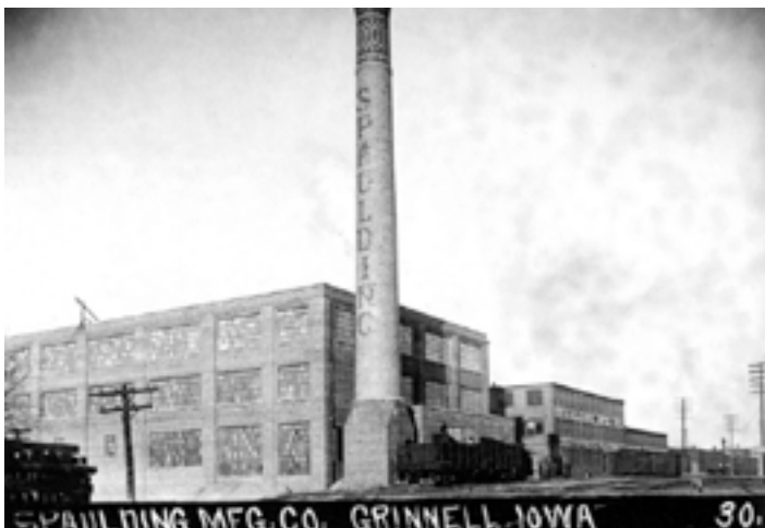
Figure 6: Spaulding Factory Building #5 from SW (Courtesy Drake Community Library)
